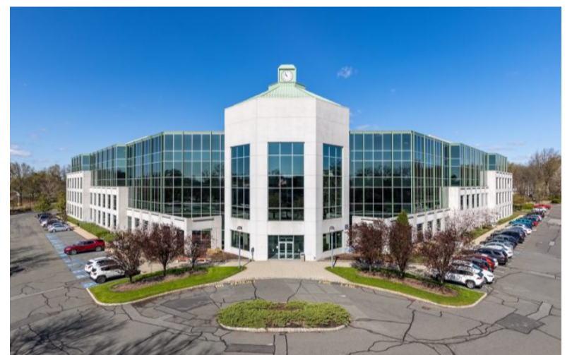
Parkway Commerce Center, 20 Commerce Drive, Clark and Cranford. – SIGNATURE ACQUISITIONS
