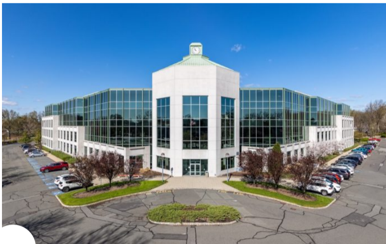
Parkway Commerce Center, 20 Commerce Drive, Clark and Cranford. – SIGNATURE ACQUISITIONS
