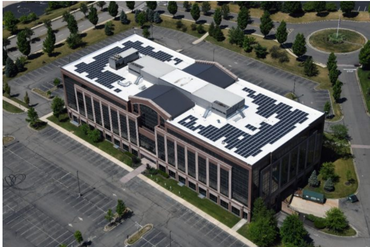
100 Kimball Drive, Parsippany. - Signature Acquisitions
