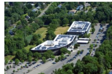
Solar energy system covering roof space across 420-430 Mountain. - Signature Acquisitions
